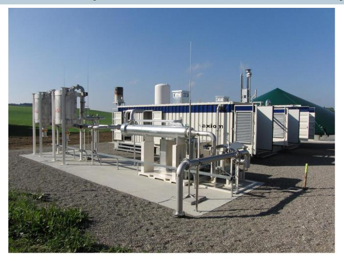
Capacity 500 m³/h biogas, 300 m³/h biomethane, approx. 8 km pipeline for grid injection and high pressure compression to 60 bar
